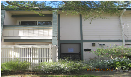
1381 Terra Nova Blvd. Pacifica, CA
